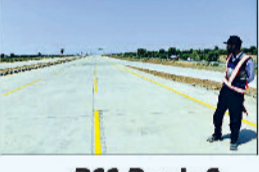
RCC Roads &amp; Wide Roads
